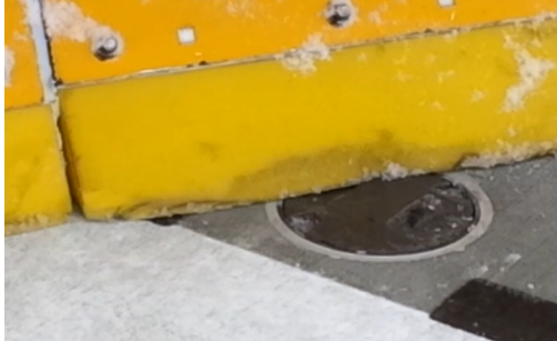
Figure 33: Fig. 3 — Snowplow blade without clearance
